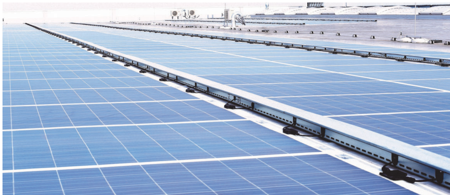
Rooftop installation DAS Energy Headquarters
